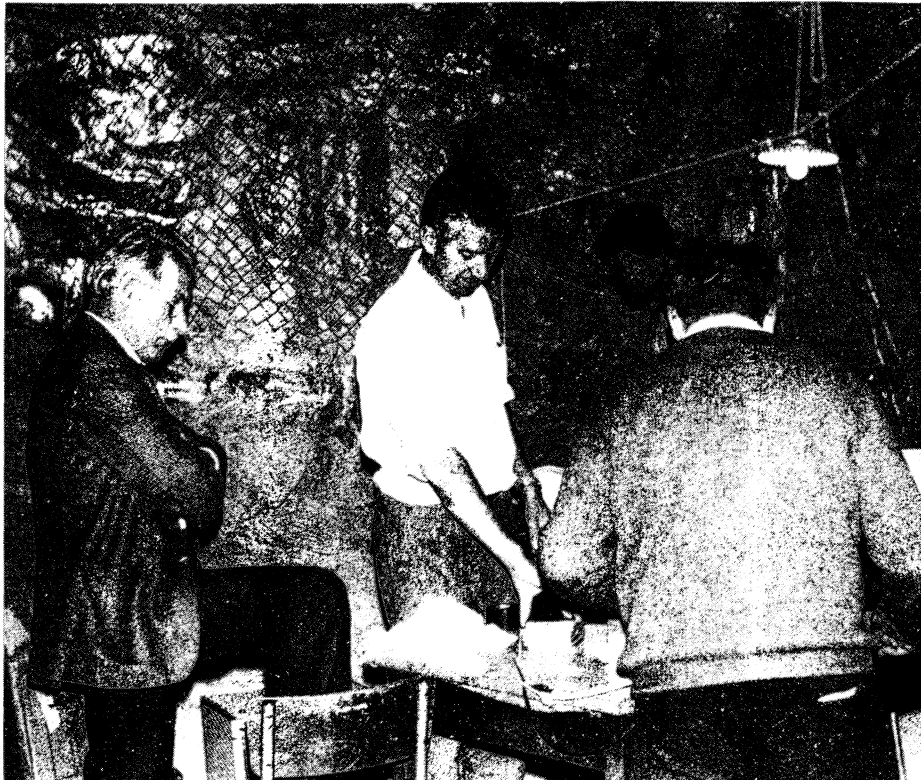
Background measurements in the initial excavation in the Fréjus tunnel.
